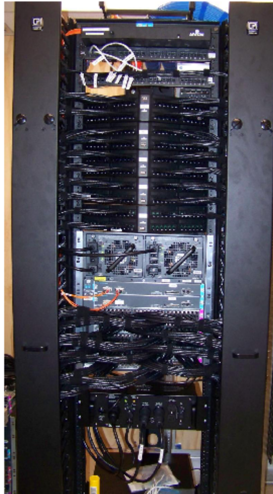
Standard Rack Design for MDF/IDF Rooms
